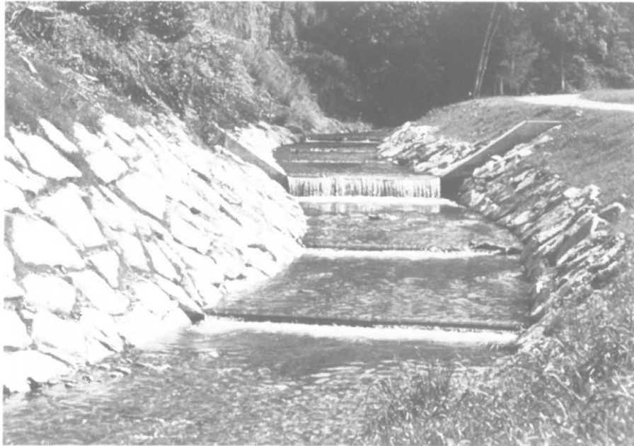
Fig. 3 Heavily trained stepped channel
