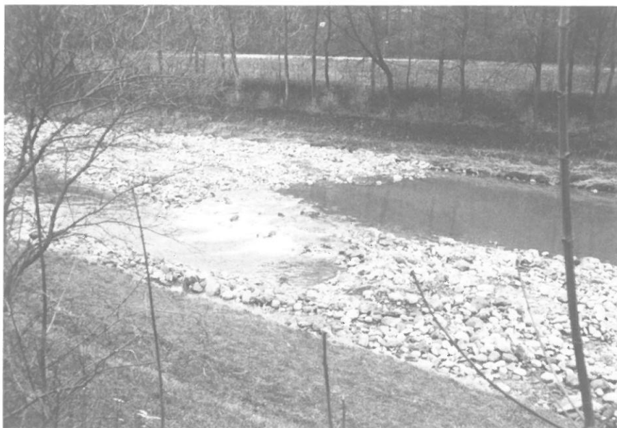
Fig. 5 Sihl river near Zurich. Low flow conditions after the bed topography has been remodelled into alternate bars.
