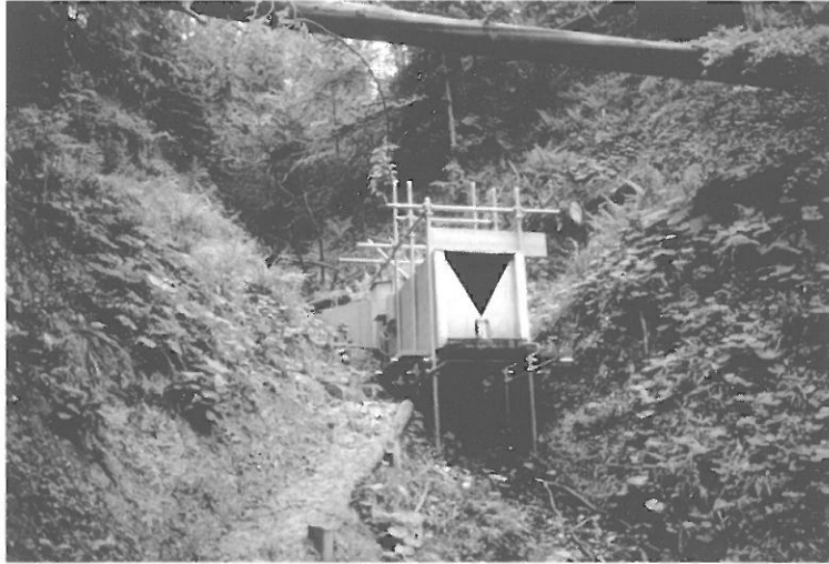
Figure 4-1: View from downstream on the gauging station at the outlet of the heavily damaged sub-catchment.
