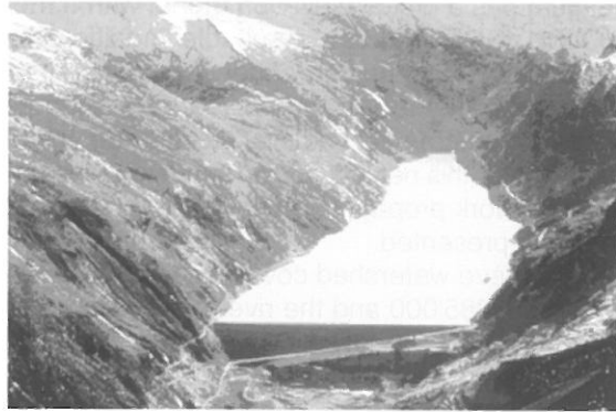
Figure 4-3: Dam of Mattmark (Switzerland).
