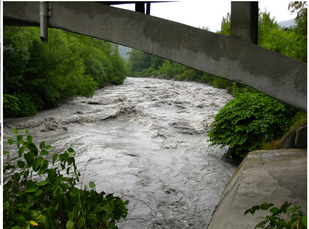
Arc River during flushing operations - June 2011
