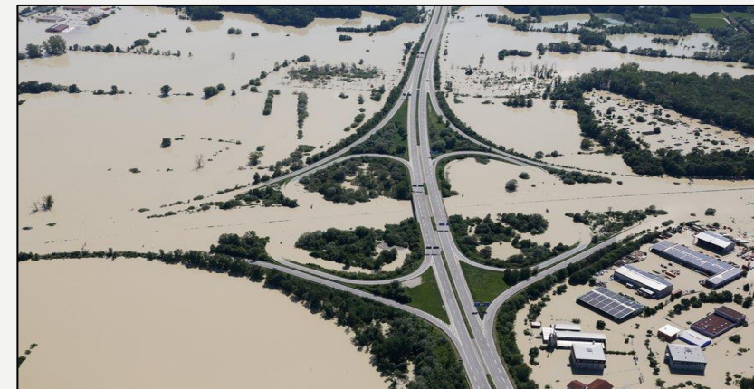
Major flood events in Bavaria 1999/2002/2005/2013/2016
